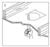
Open the ceiling to be mounted in accordance with the downlight cutting diameter you have selected.
